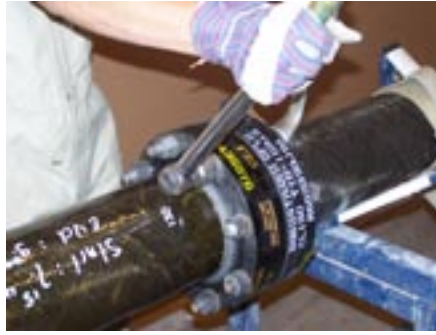
Photo 21 - Tighten bolts
