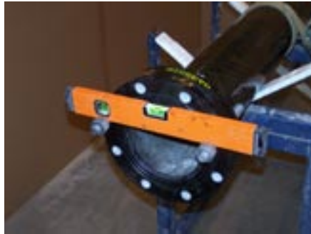
Photo 7 - Check bolt holes alignment
