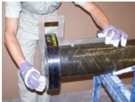
Photo 9 - Check alignment of flange face
