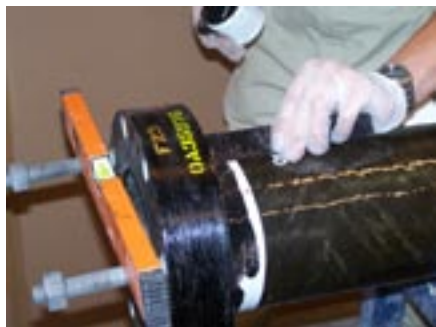
Photo 10 - Remove excessive adhesive
