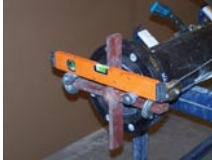
Photo 17 - Check alignment of bolt holes
