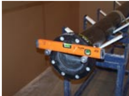
Photo 14 - Check boltholes alignment
