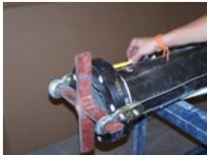
Photo 15 - Check insertion depth
