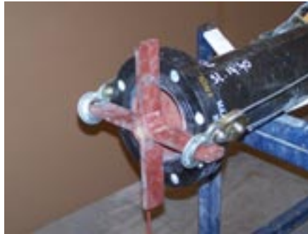
Photo 18 - Cure the adhesive joint
