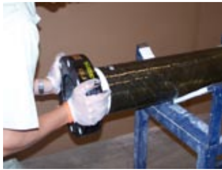
Photo 6 - Push flange onto spigot
